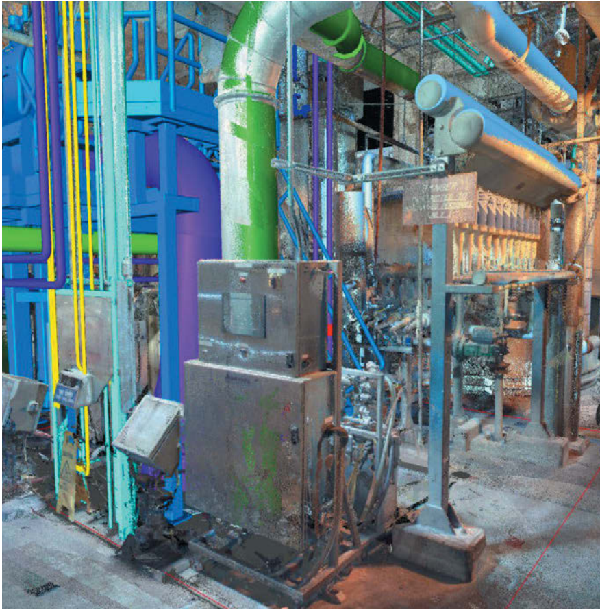
For Project 2, the 3D fabrication model was overlaid on the laser scan.
