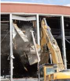
Crews stripped the facade from the Brown County Veterans Memorial Arena on July 9, 2019 (Photo: Richard Ryman/USA TODAY NETWORK-Wisconsin)
